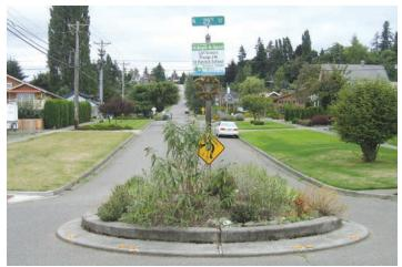
Figure 4.27: Mini Roundabout, Source www.pedbikeimages.org, Photo - Carl Sundstrom
