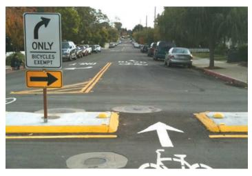
Figure 4.16: Diverter, Source www.pedbikeimages.org, Photo – Adam Fukushima
