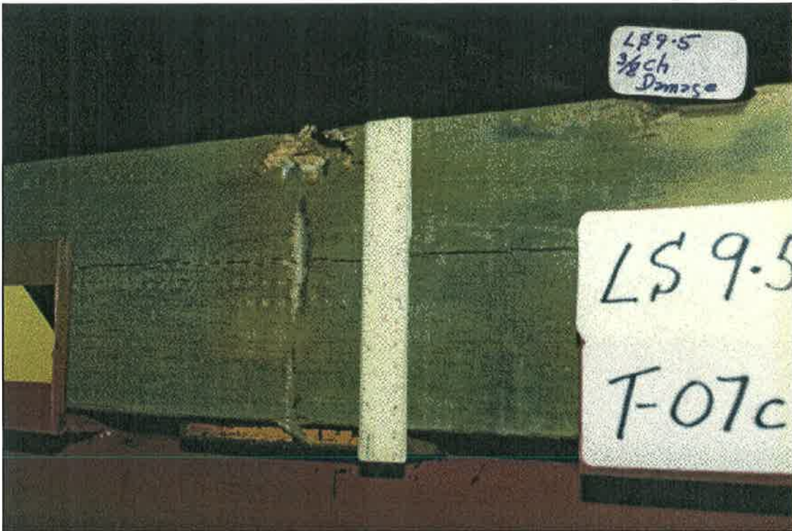
Figure 15/ Damage to Spruce by Chain Tiedown
